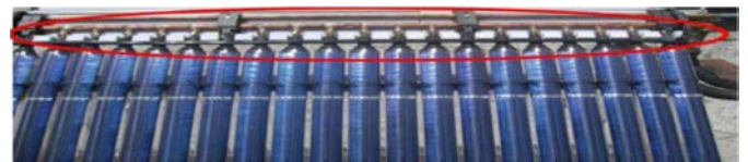
Figure 1. Circulation pipe of evacuated tube collector
